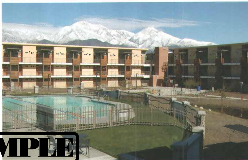
AT THE END of its three-phase Residential Life Project, Pitzer College expects to become the first in the nation to boast all gold-LEED-certified residence halls.
